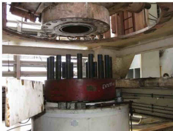
Figure 6.1: Installing the Cameron HC Collet Connector
