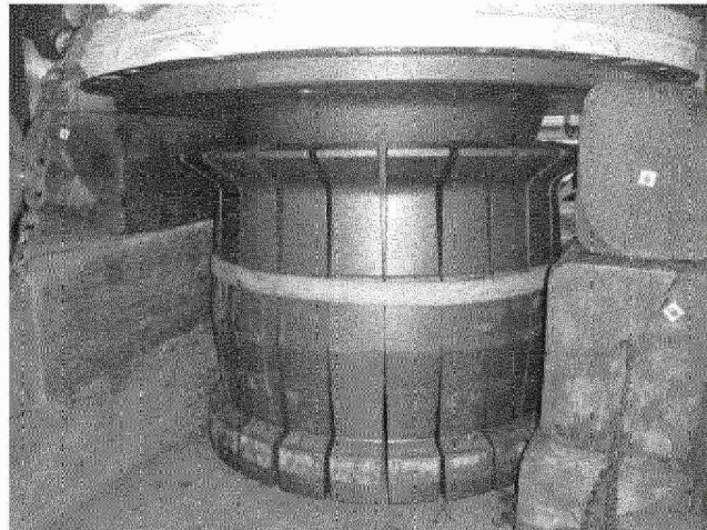
Figure 5.3: Shows the body section removed with collets secured to hub.
