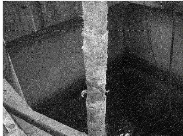
Figure 2: Damaged outer sheath on the moonpool hose.
