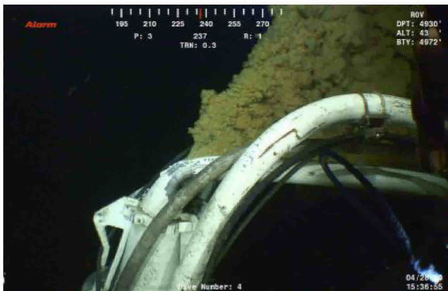
Figure 4. Photograph of leaks in kinked riser, taken April 28, 2010.
