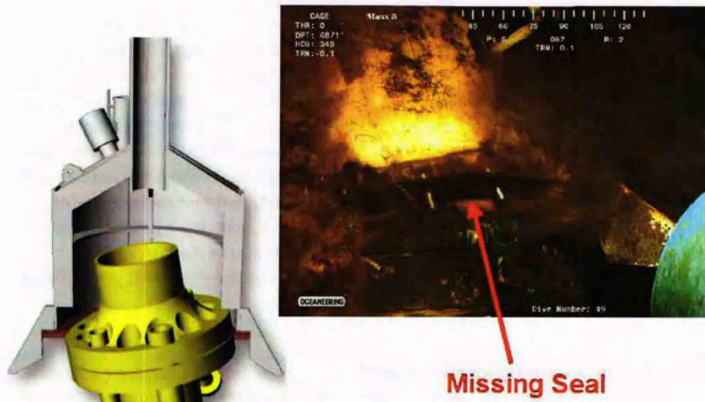
Fig. 7: Image of Top Hat over Riser With Missing Seal
