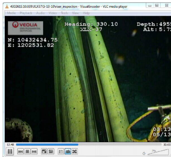
Figure 1 – Screen capture of XLX-37 Riser Survey video on May 13, 2010
