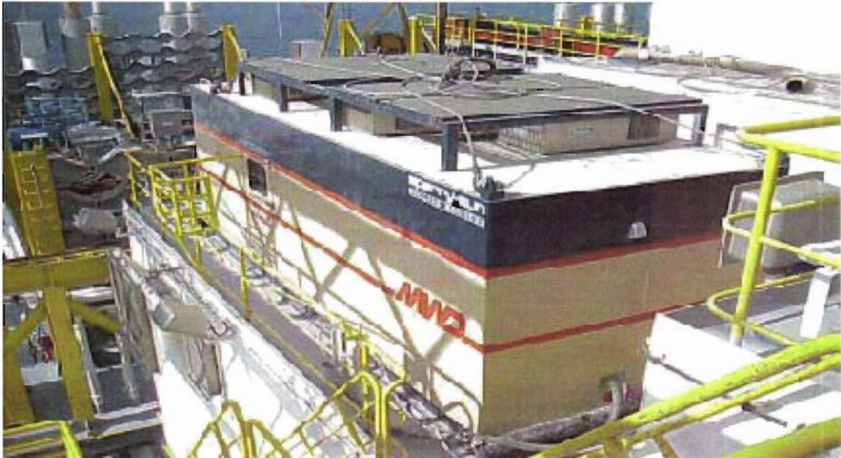
Figure 21: A Mudlogging “shack” on the Deepwater Horizon circa 2003 36
