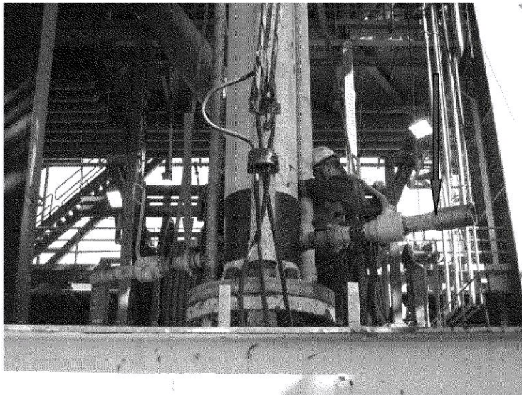
Figure 12.2: ROV operated ball valves (red arrows) installed and MUX cables installed on the riser joint.
